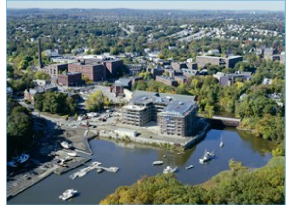
The Residences at Milton Landing, Source: miltonlanding.com
