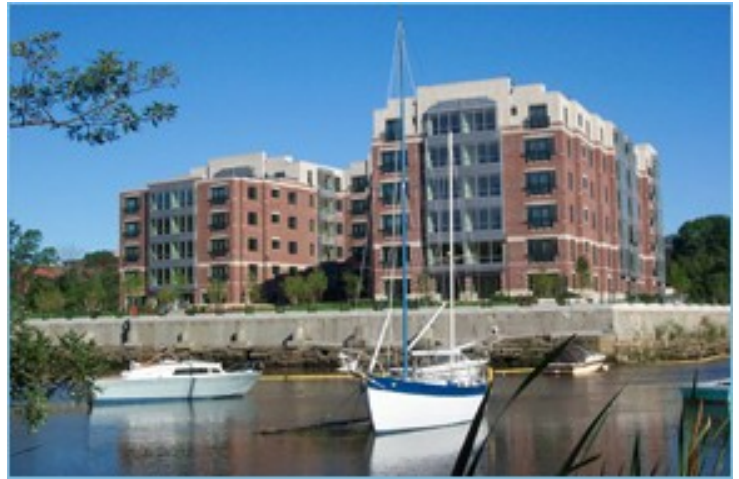
The Residences at Milton Landing, Source: miltonlanding.com
