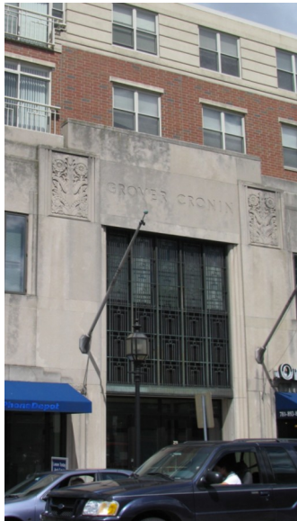
The original Grover Cronin's storefront façade, 2010.
