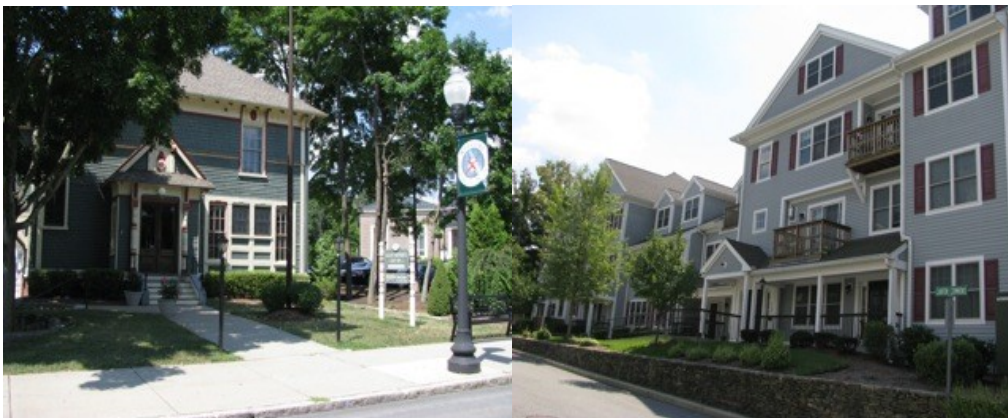
Grover Estates: Historic preservation and new townhouses, 2010.
